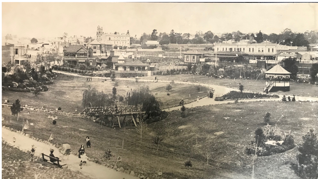
Canterbury Gardens looking east towards Maling Rd and the railway c 1910. (CHG)
