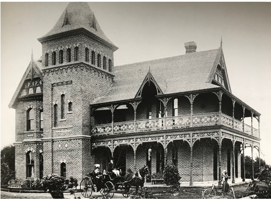
L: 'Tourmont', later Fintona, showing decorative brickwork, gabled slate roof and fine lacework of the return verandahs. Family members are seated in the carriage.
